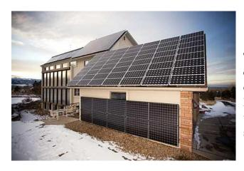
This homeowner has placed panels on almost every flat, exterior surface of their home. The ones on the roof may be at a good slope. However, the ones on the garage doors are vertical. They would not be useful when the sun is positioned overhead.
